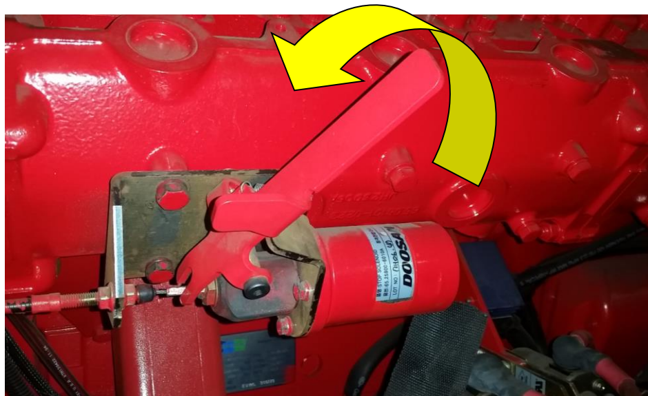
Figure 4e – DR8H, DS0H manual stop override lever located at front of engine, above belt guard;
